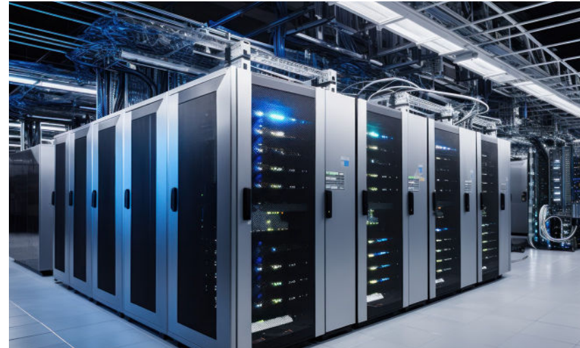
Server racks in a data center
